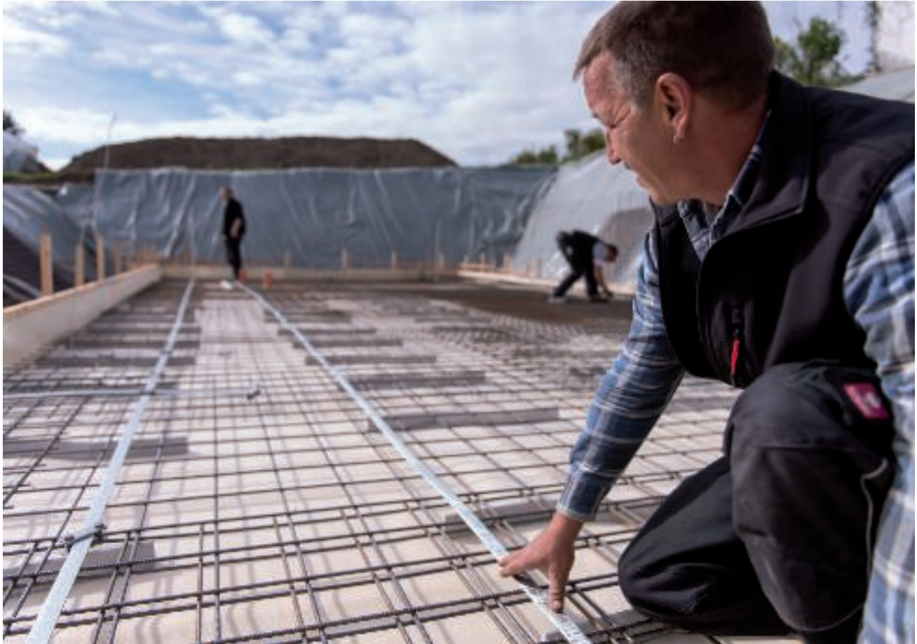
Installing a foundation earther
