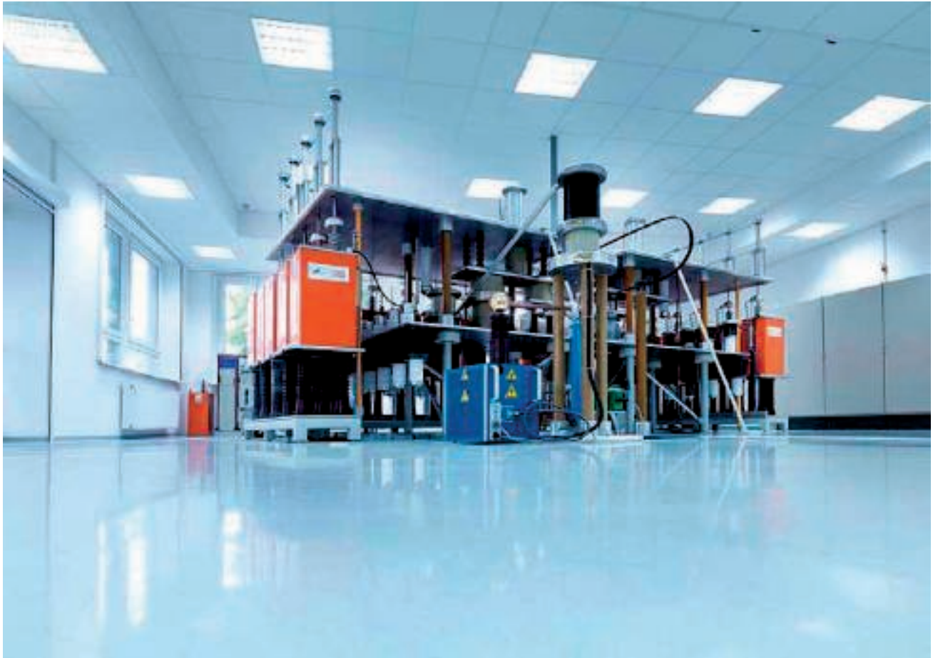
Lightning current generator
